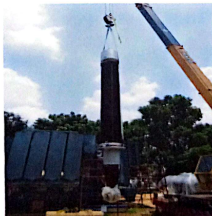
Gambar 2.19 Instalasi Bushing
